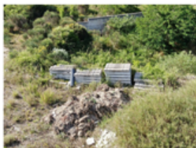
2. TRAVERSINE E RESIDUI IN CALCESTRUZZO
